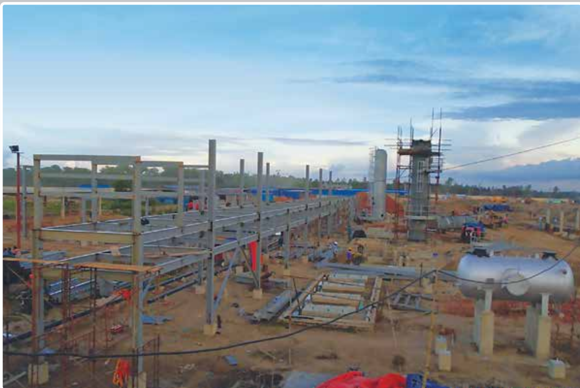
Equipment, Vessel, Piperack Installation.
